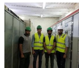
Energy Audit of Electric Panels
